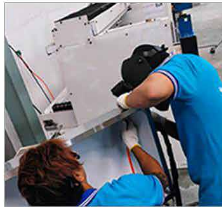
Thai workers doing the welding
