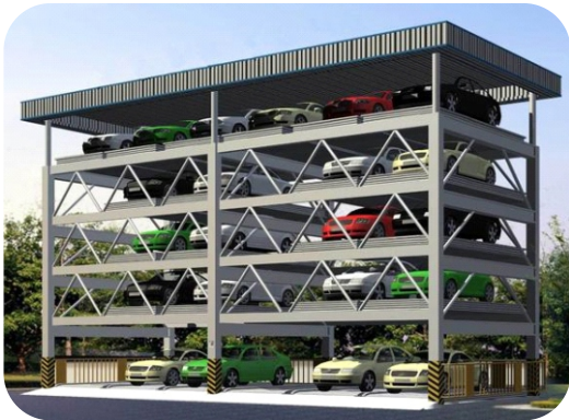
Automated parking system
