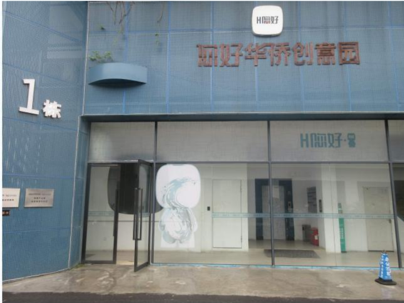
Company Building Gate
