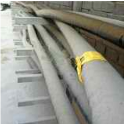
marks are accurately distributed to each cable
