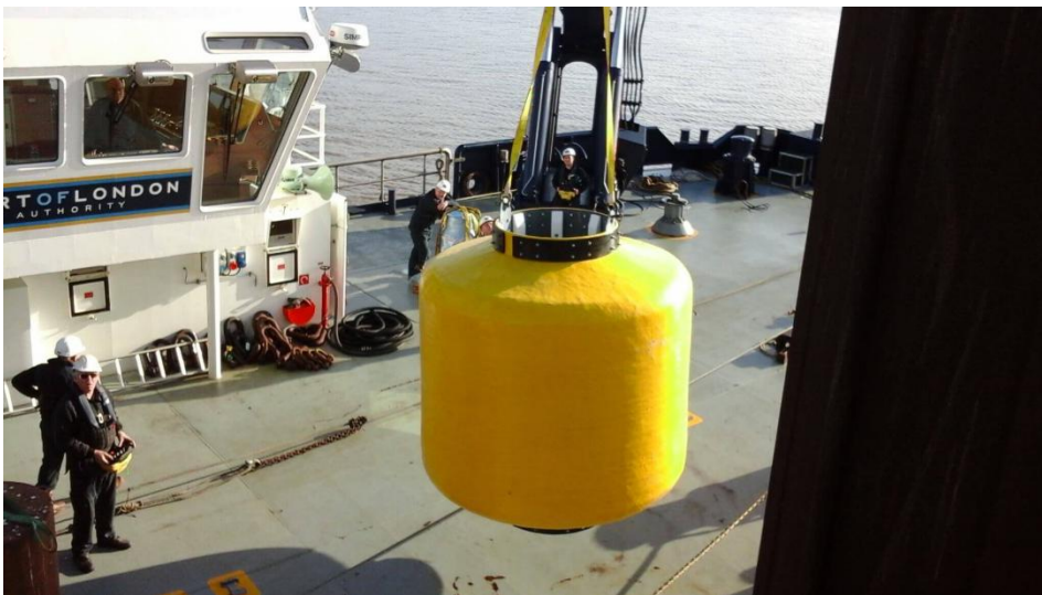
Installation of donut fender
