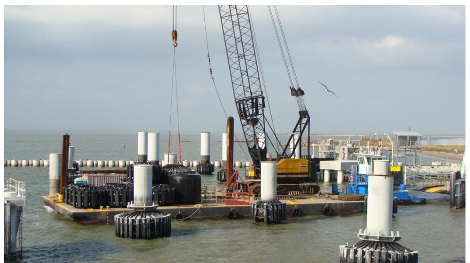
Donut fender with protective cover
