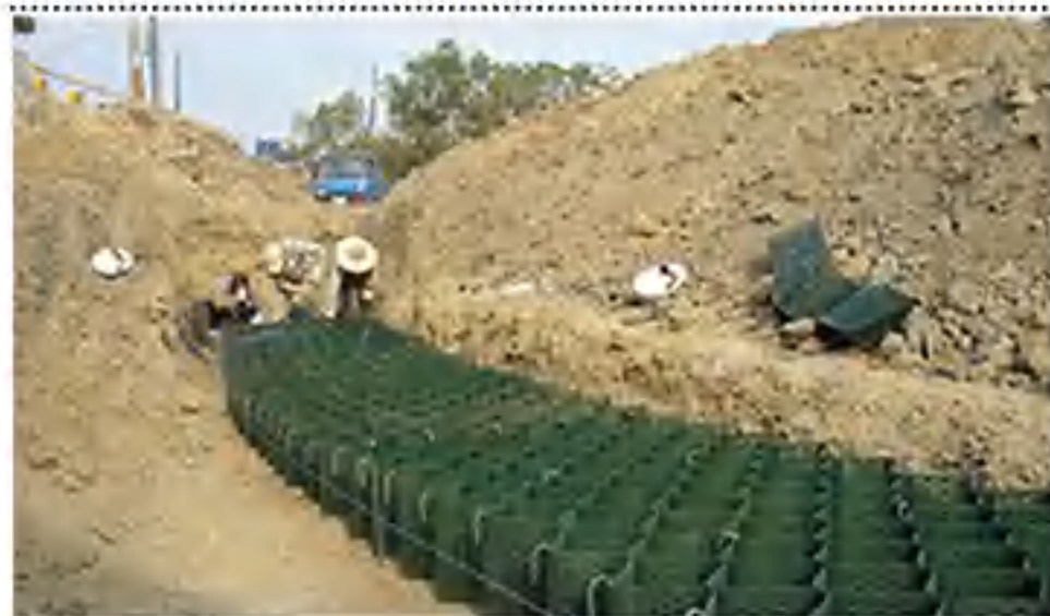
Plastic Gravel Stabilizer Geocell
