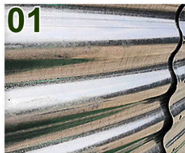
01 Sheets are connected end to end
