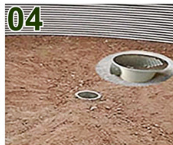
04 A slope for centralized drainage
