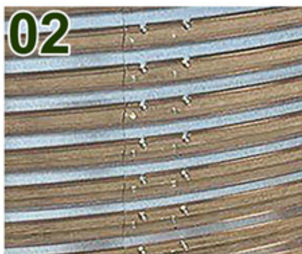
02 Connect and tighten Screws
