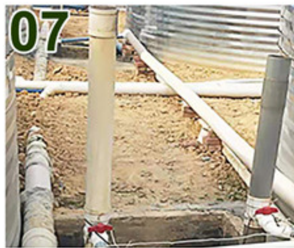
07 Connect to the outside water outlet
