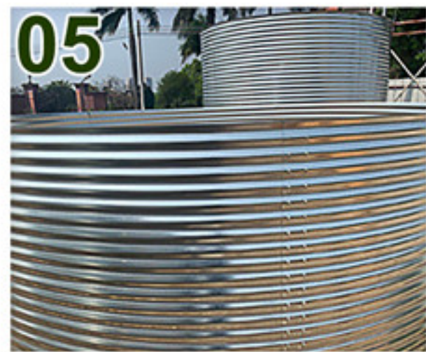
05 Installation of the galvanized sheet
