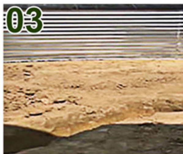
03 The bottom is made as a buried pipe
