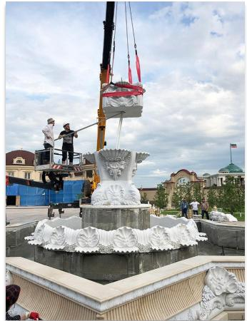
According to the drawing number, find the center point of the fountain, install it gradually from bottom to top, and ensure the level of stone.
