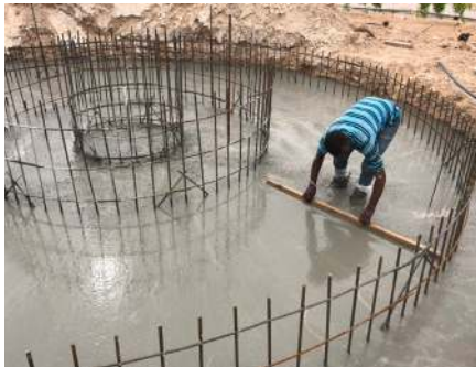
01. Concrete foundation construction
