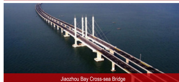
Jiaozhou Bay Cross-sea Bridge
