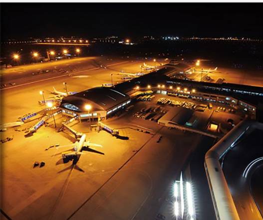
Carbon Steel Pipe used in Beijing Capital International Airport
