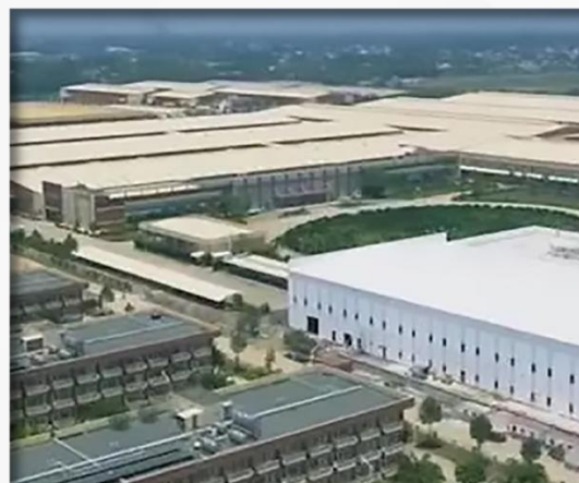
Solar mounting systems steel pipe used in Cong ty TNHH Gain Lucky Textile Factory Vietnam
