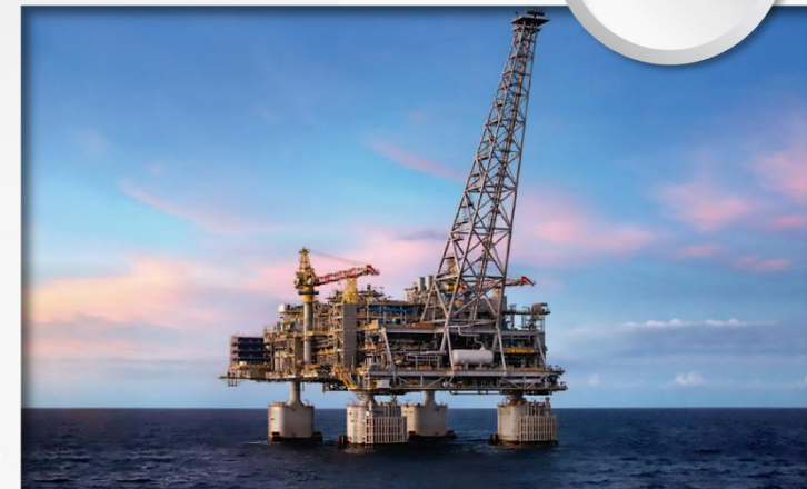
Scaffolding Steel Pipes used in Chevron Corporation Oil Platform
