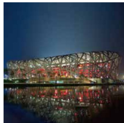
Construction Steel Pipe used in Beijing National Stadium-Bird's Nest
