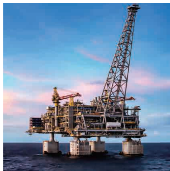
Scaffolding Steel Pipes used in Chevron Corporation Oil Platform
