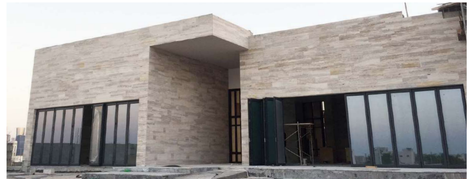
- Folding Door Installation
