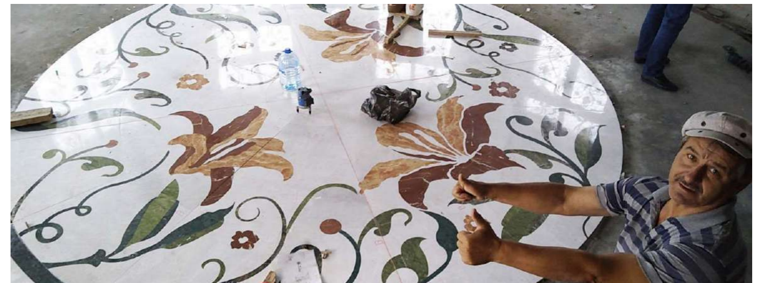
-Under Installation By PFM Team
