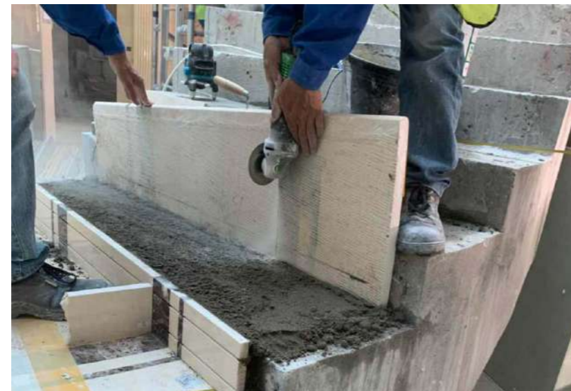
- Under Installation By PFM Team
