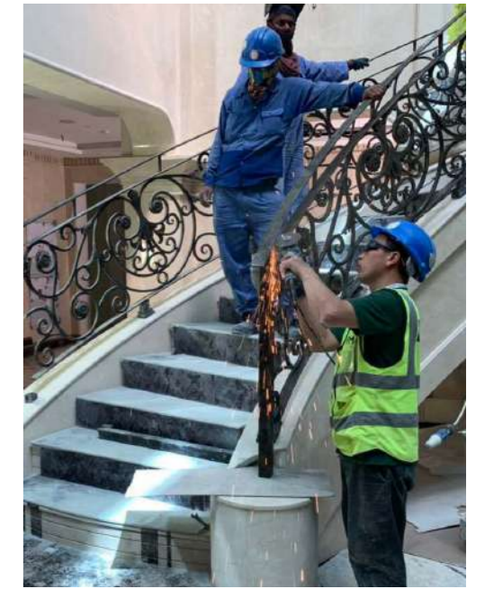
- Under Installation By PFM Team
