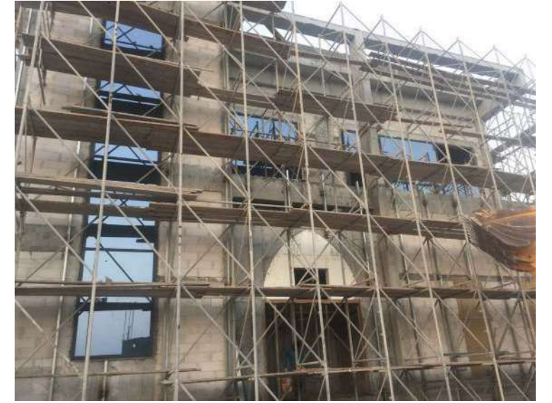
- External wall and window installation
