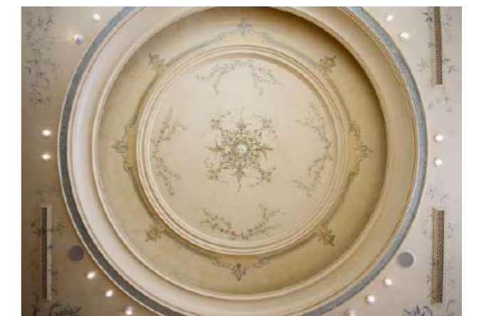
-Living Room Ceiling
