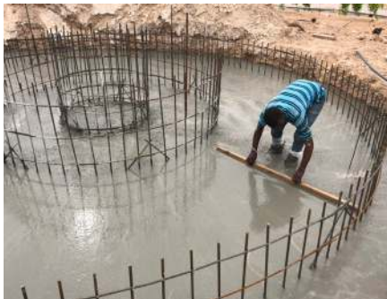
01. Concrete foundation construction
