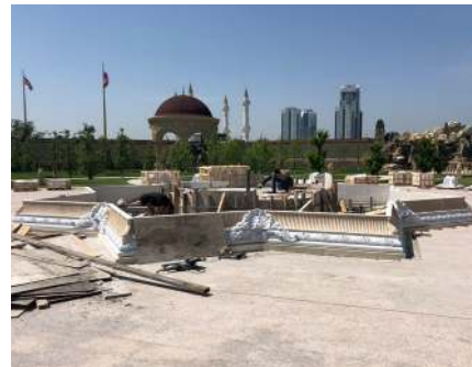
03. Surrounding pool installation
