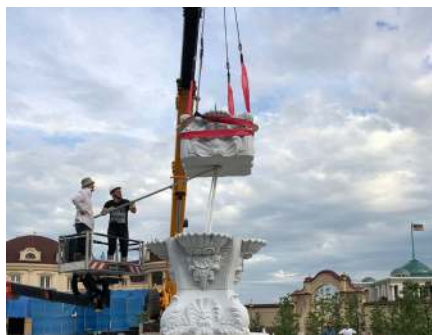
05. Preassembling with crane
