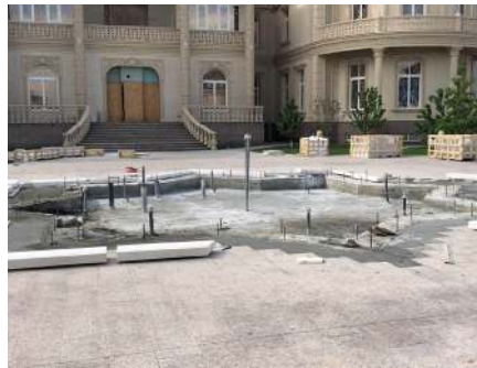
02. Water supply system installation
