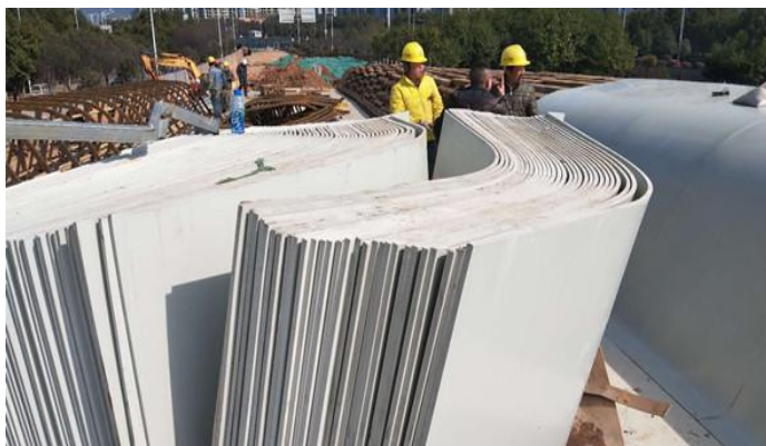
Concrete Formwork For Bridge
