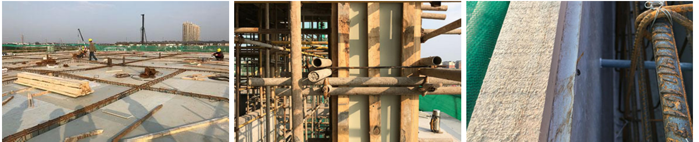
Art Museum (using fair-faced pvc concrete formwork)
