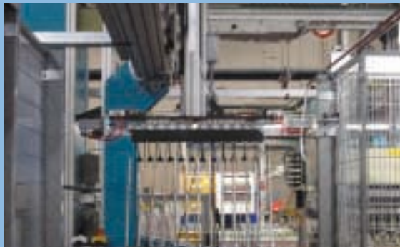
The robot, controlled by two Beckhoff servoamplifiers, installs the cables within the spray lines.
