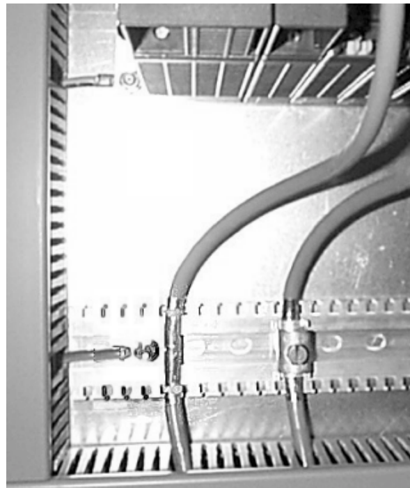
This is an example of earthing internal shielded cables. 2 solutions are shown here, one with a metallic fastening.
