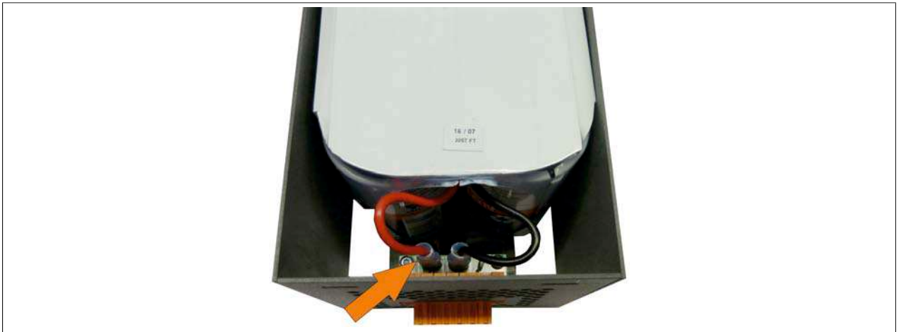
Figure 211: Disconnecting the cable
