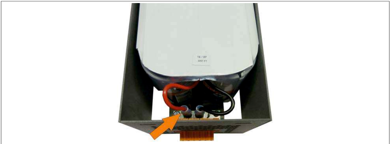
Figure 212: Disconnecting the cable
