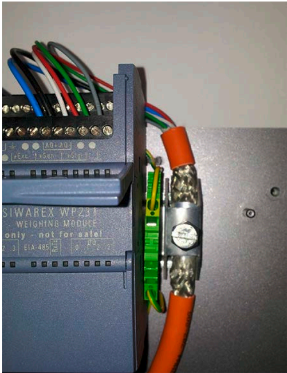
Image 6-3 Installation of the shield connection element (example)
