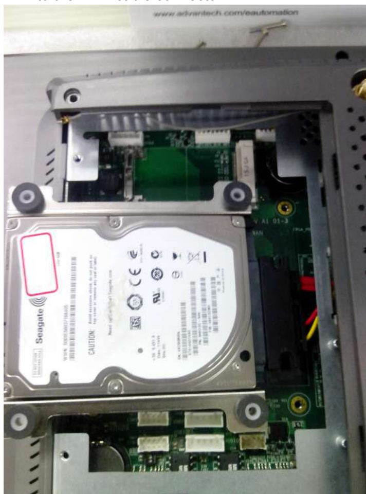
Figure C.4 Connecting the HDD cable
