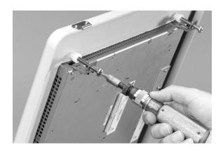
7. Alternately tighten the mounting clips screws to a torque of .90 - 1.1 N•m (8 - 10 in-lb). Do not over-tighten.
