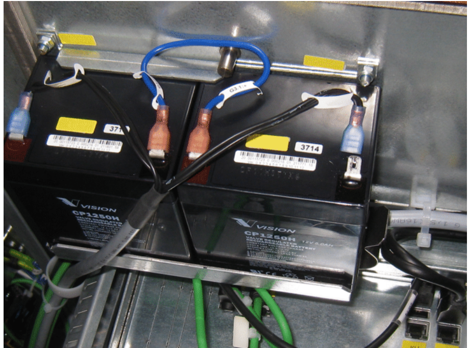
Fig. 11-32: Battery fastening in the cabinet door
