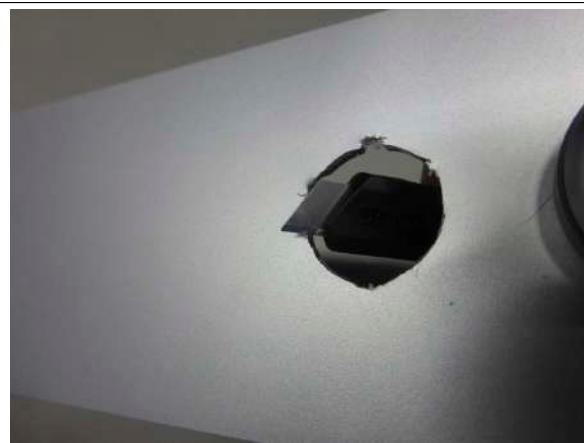
Figure 85: Cutting the panel overlay so it is flush
