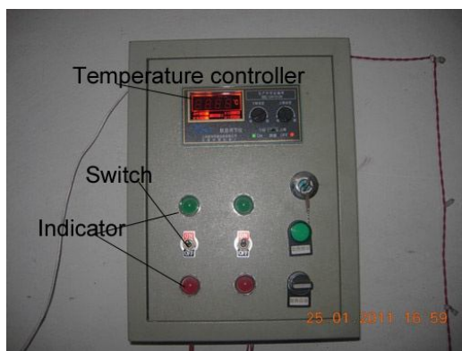
Electric Cabinet/Thermostat
