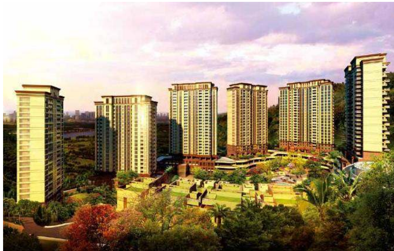
7 The Landcom Hill Manor, Shenzhen
