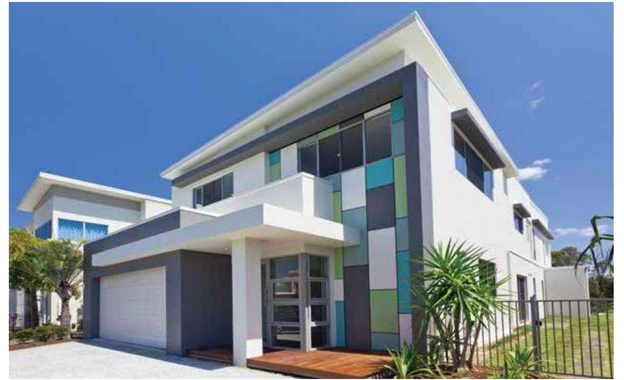
↗ Vanke Jiulong Mountain Villa, Shenzhen
